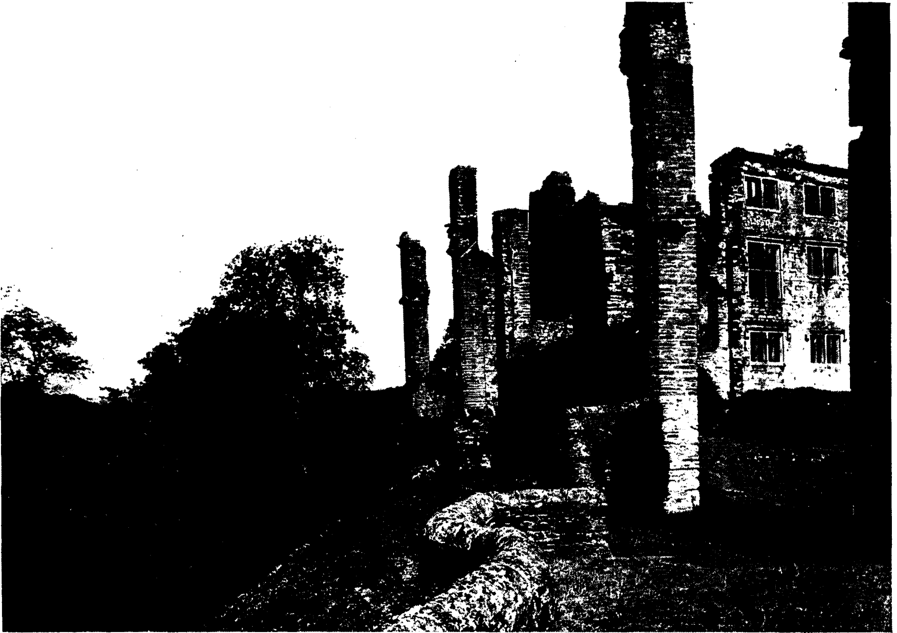
ALONG THE NORTH SIDE: SEYMOUR BUILDING
