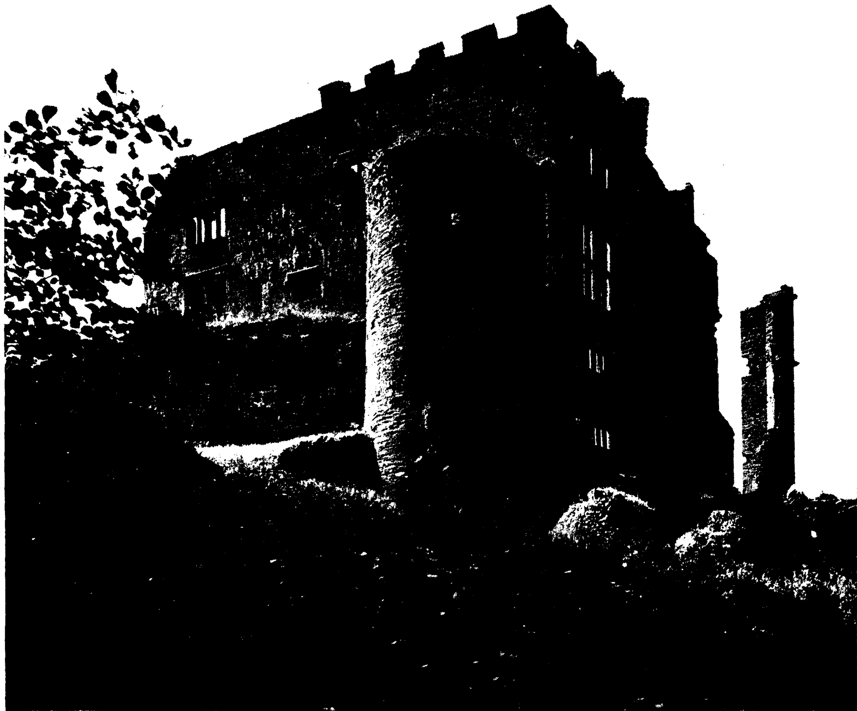
FROM THE SOUTH-EAST CORNER: ST MARGARET'S TOWER AND SEYMOUR BLOCK
