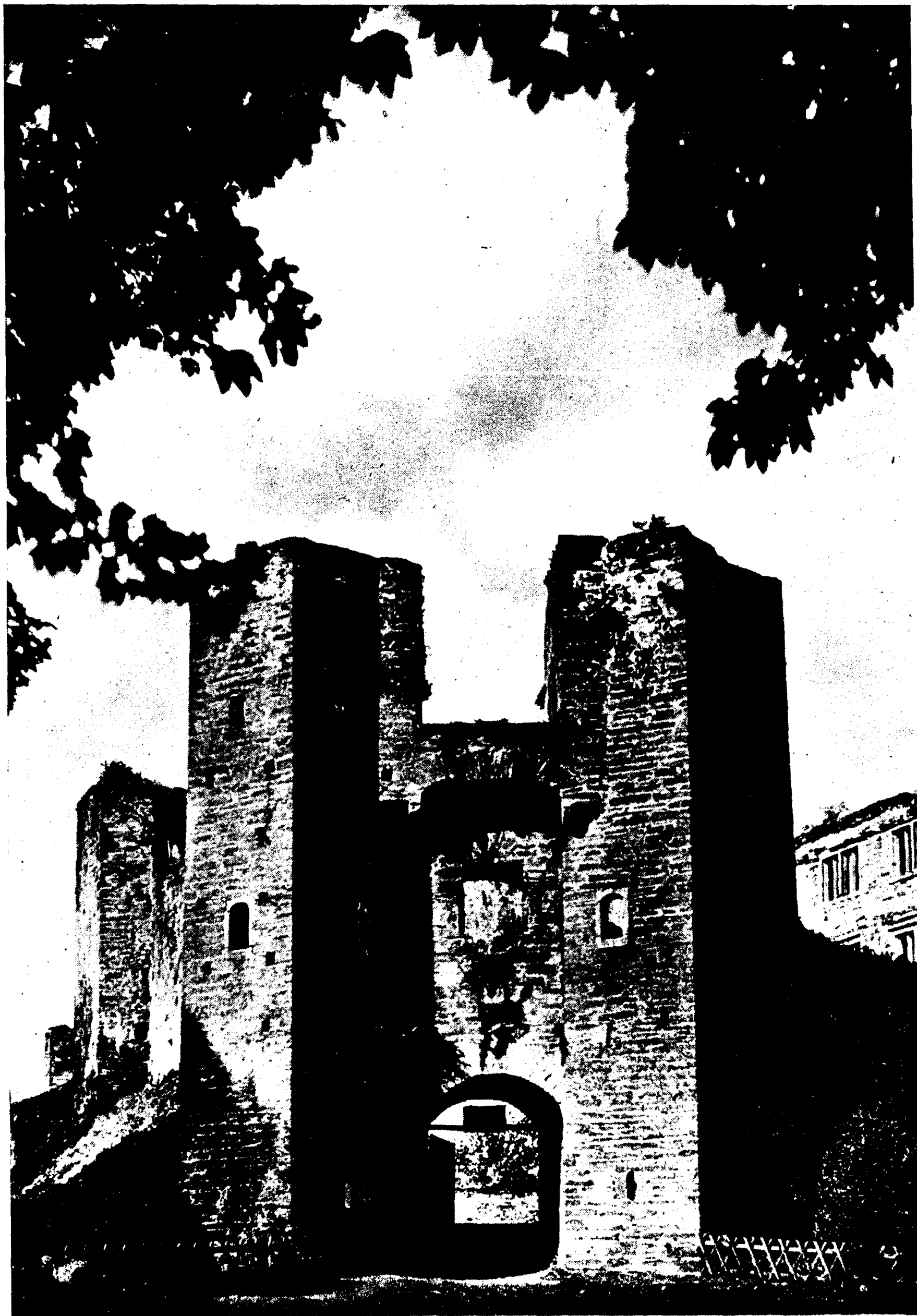
GATEHOUSE AND FLANKING TOWERS
